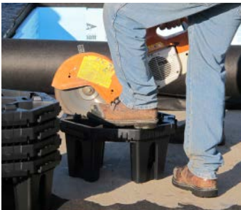
StrataCell being customised and cut in half to fit tight below underground constraints.
