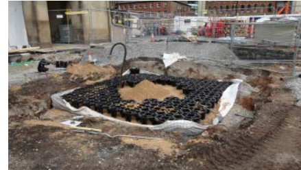
GreenBlue Urban's StrataCell soil cells were used to provide these trees with quality, uncompacted soil.
