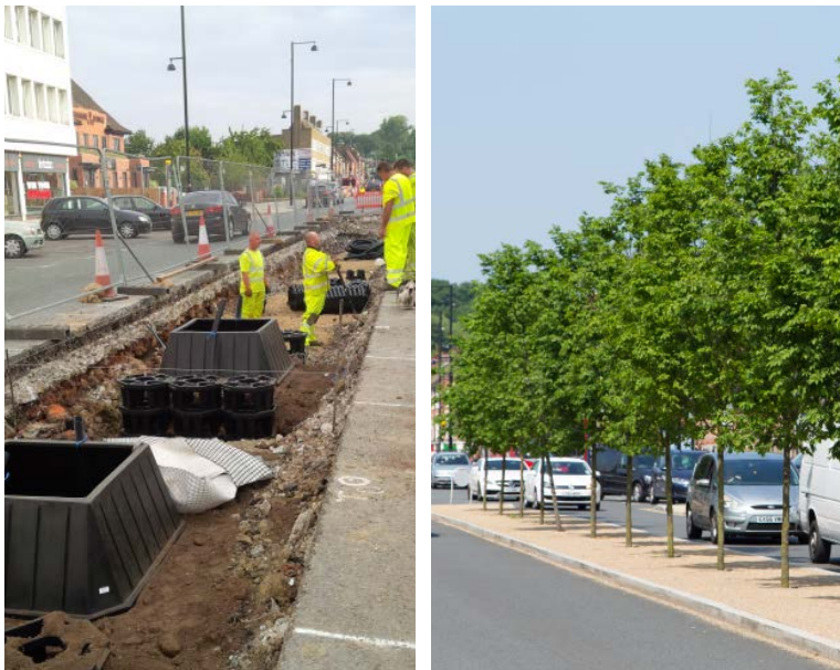
RootDirectors are the ideal root management solution for individual tree planting schemes, and were used in both the above projects. Used here in a project in Northwood Hills, Hillingdon, London.
