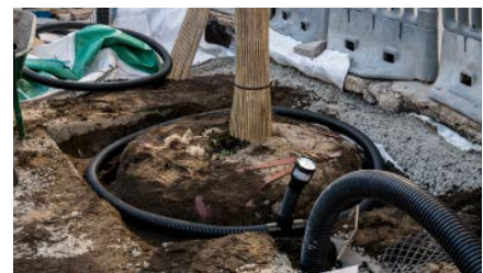
RootRain Civics around the Rootball and ArborVent's with custom brass grilles were included to ensure the soil stays aerobic.
