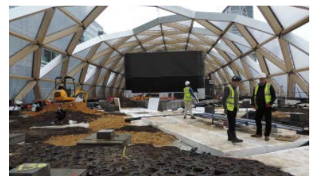
Root barrier was used around the perimeter of the StrataCell matrix in order too effectively manage tree roots.
