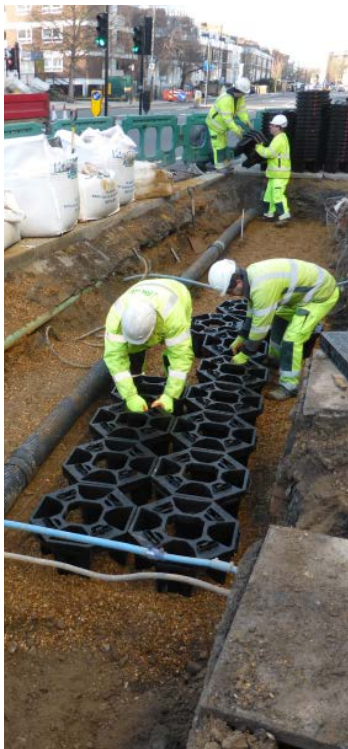
Installation of the StrataCell tree pit on Goldhawk Road.
