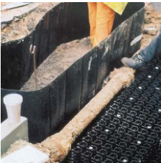
ReRoot 1000 installed to protect underground services and divert roots beneath pavement surfaces into the preferred rooting area.
