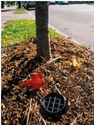
This illustrates the correct level for the RootRain Urban inlet. Too low could lead to blockages; too high can look obtrusive.
