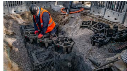
A combination of StrataCell and RootSpace were used to provide uncompacted soil volume whilst working around busy services and other site constraints.
