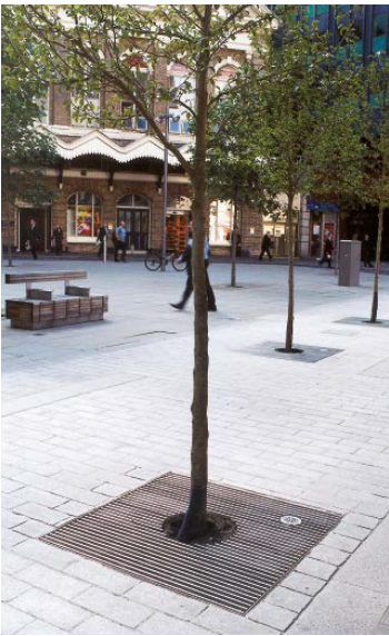
'Clyde' grille, in central London, manufactured from grade 316 stainless steel.
