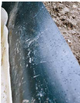
ReRoot 2000/RootStop will hold its form in a trench excavation. This makes installation quick and easy. Also visible is land drain to remove groundwater pressure.
