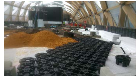
StrataCells were specified in order to provide trees and plants quality uncompacted soil medium.
