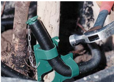
Nail the bracket to the tree stake before backfilling to conceal the Metro bracket.
