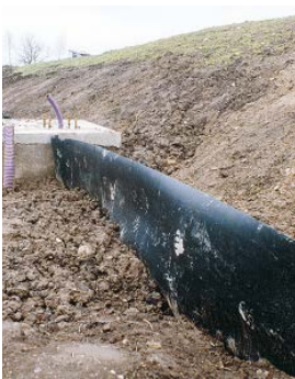
ReRoot 2000/RootStop has been installed prior to topsoiling in this infrastructure project.
