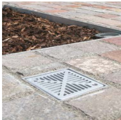
RootRain ArborVent inlet set in paved surround.
