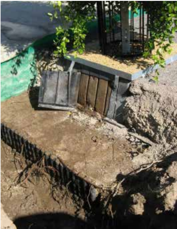
Modular root barriers direct roots slightly downward and outwards to protect paved surfaces
