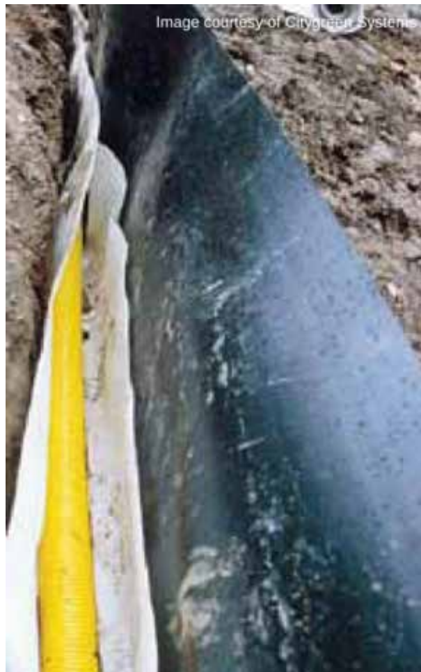
Smooth linear barrier laid along utilities
