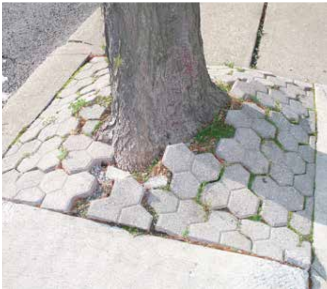
Using a RootDirector would have guided root growth to lower depths which would have prevented this upheave at the base of the tree
