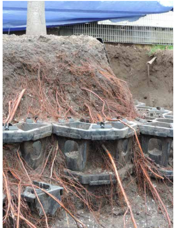
Modular root barriers direct roots slightly downward and outwards to protect paved surfaces
