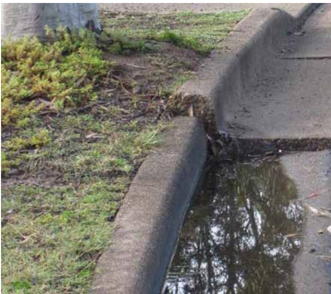
This unmanaged root system has lifted the curb and created a drainage issue
