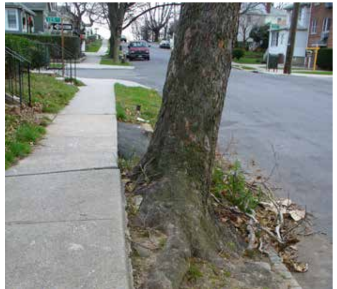
Tree roots lifting and cracking the sidewalk, a common sight in urban areas.
