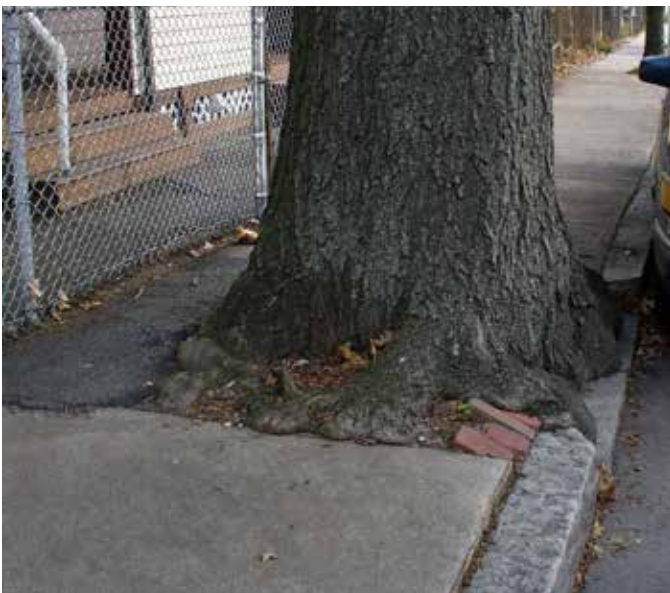
There isn't much that can be said for this situation Mature trees are not easily dealt with when they reach conditions like this
